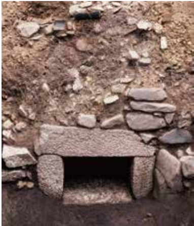
5 Bakuro-cho Kamigyo-ku (precinct of Kitano Tenmangu Shrine) Stone-built culvert outlet
